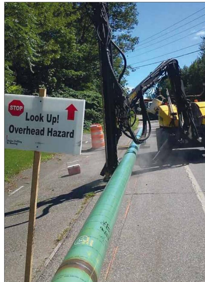
Probing on the Summit Natural Gas Pipeline, Maine, to identify rock removal needs.
