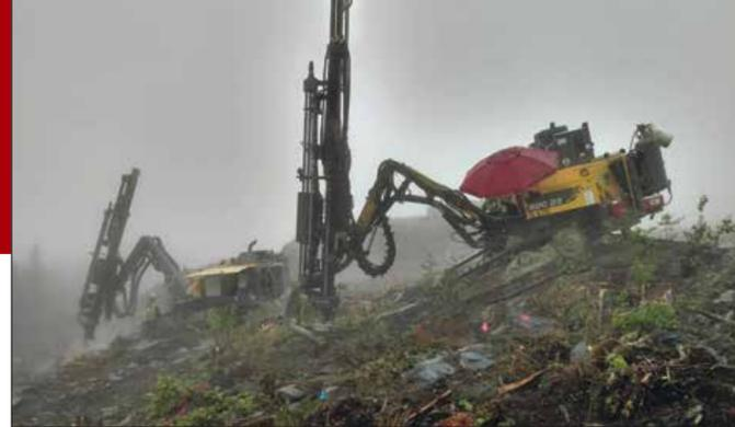
Drilling for rock removal on access roads and for wind turbine pads on Maine's Bingham Wind Farm.
