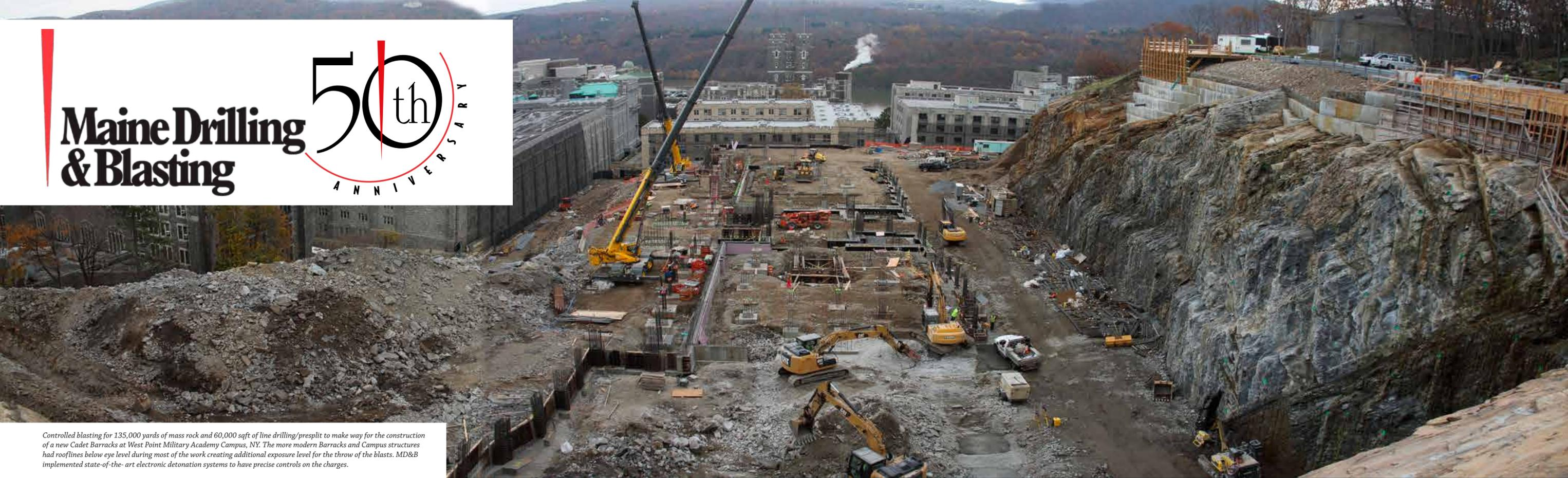
Controlled blasting for 135,000 yards of mass rock and 60,000 sqft of line drilling/presplit to make way for the construction of a new Cadet Barracks at West Point Military Academy Campus, NY. The more modern Barracks and Campus structures had rooflines below eye level during most of the work creating additional exposure level for the throw of the blasts. MD&B implemented state-of-the-art electronic detonation systems to have precise controls on the charges.
